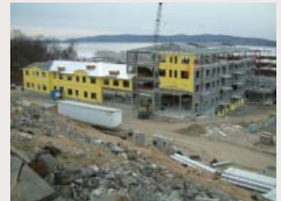
Kendal on Hudson commons building takes shape.
